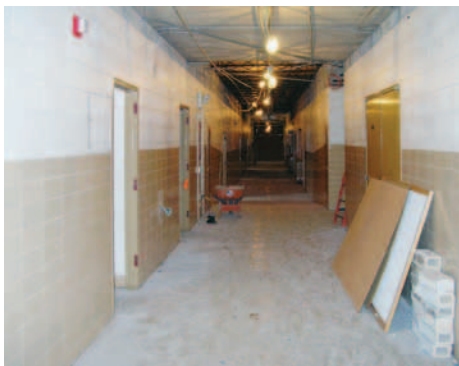
Before renovation of the new Administrative Offices and Preschool/Education building.
